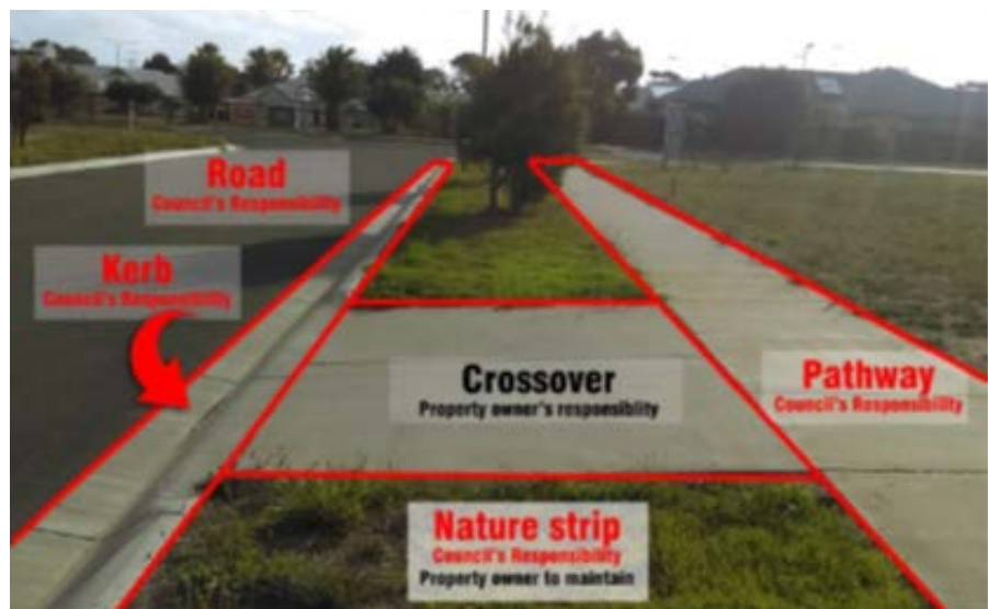
Figure 3 - Typical Vehicle Crossing Layout (Urban)
