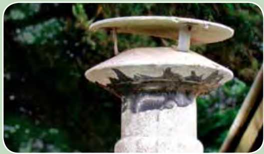
Asbestos cement flue and cowl
