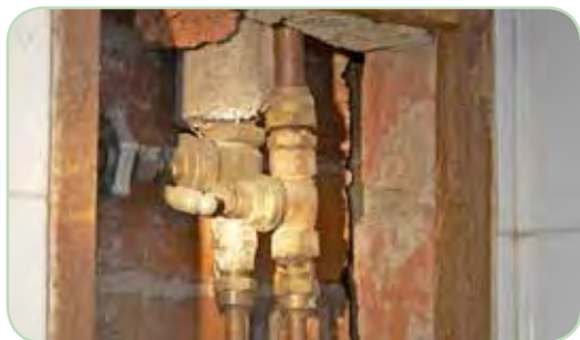
Friable asbestos lagging on pipes
