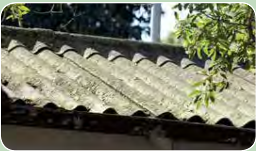
Asbestos cement corrugated roofing
