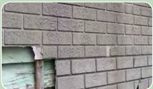
Asbestos cement 'brick' cladding
