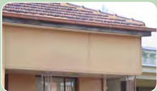
Asbestos cement sheeting in eaves
