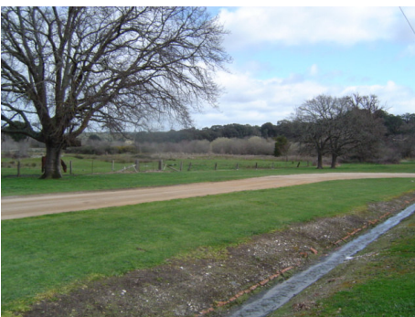
Open stormwater drain
