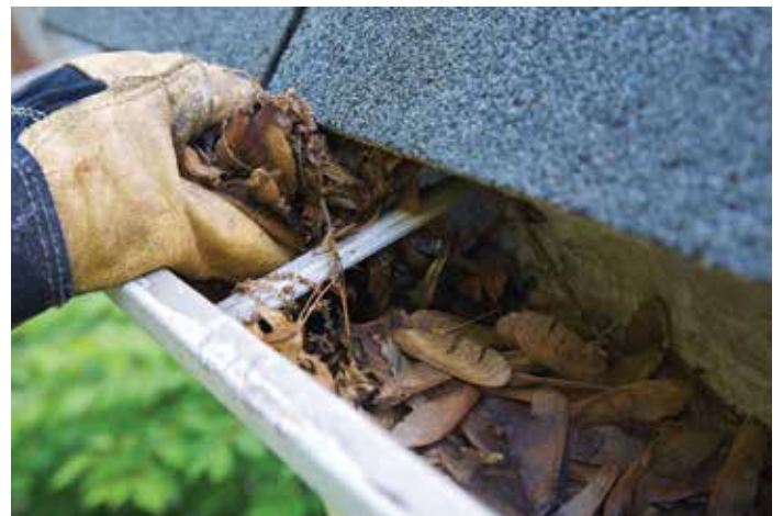
Cleaning gutters as a fire prevention.
