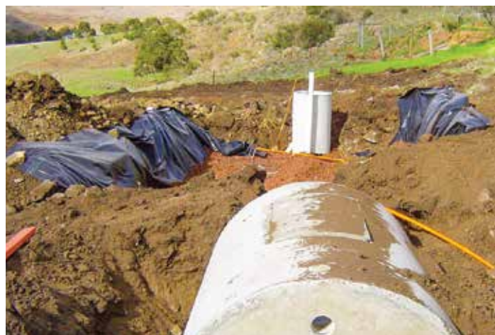
Septic Tank system being installed.
