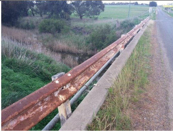
Photo 1: Barwon Park Bridge Barrier.
