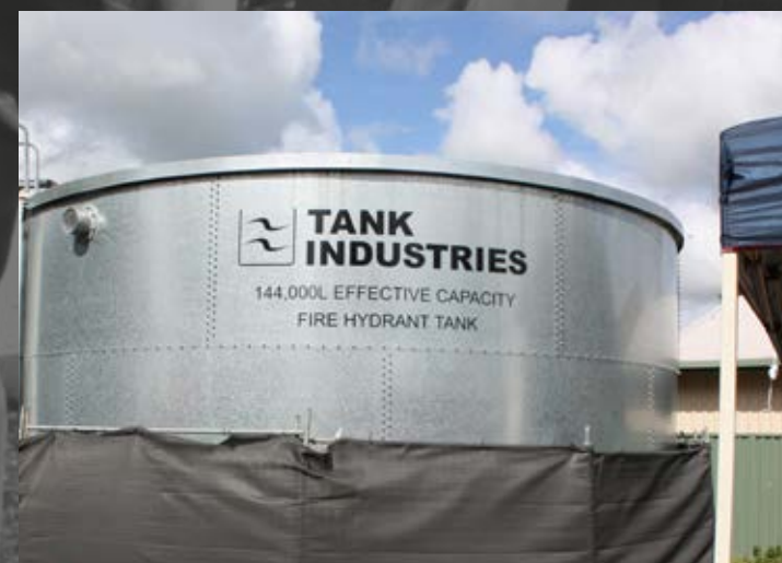
Two 144,000L water tanks are located on the site. Their purpose is to provide fire protection to the Bannockburn Cultural Centre.
