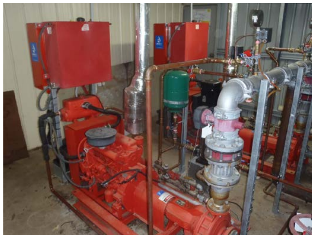
Photo No. 1: dual diesel fire pumps
