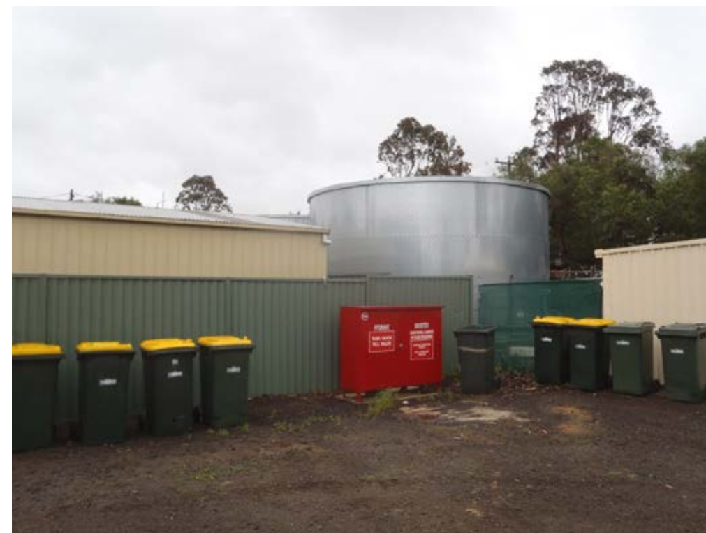
Photo No. 3: hydrant booster connection
