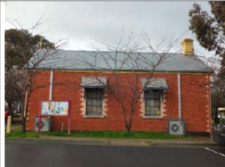
Photo 8: Rear (west) elevation. Source: David Rowe.
