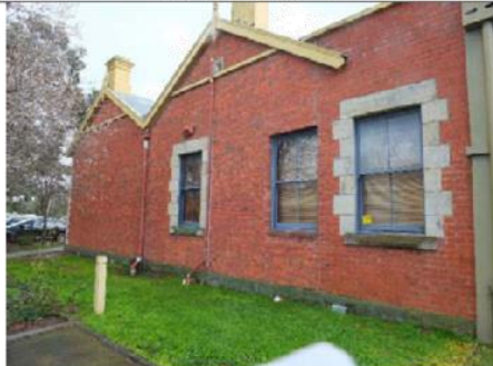
Photo 7: South elevation showing extension of 1915-16 (right). Source: David Rowe.
