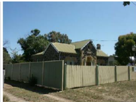
Photo 23: Former Meredith Shire Office, 2012. Source: David Rowe.
