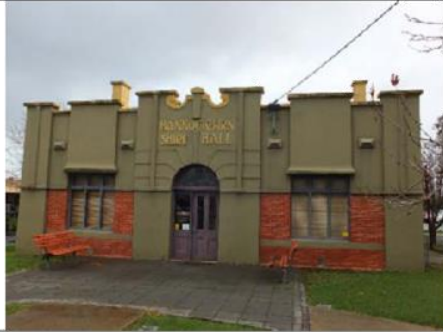
Photo 1: East (front) elevation. Source: David Rowe.
