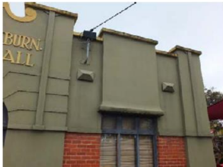
Photo 3: Detail of north bay, east elevation. Source: David Rowe.
