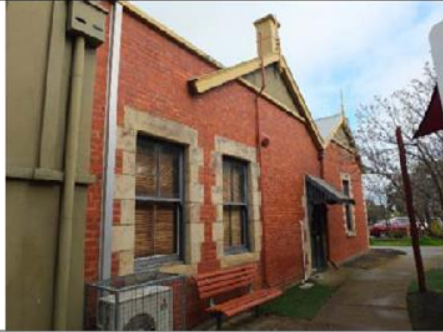
Photo 5: North elevation looking west. Source: David Rowe.
