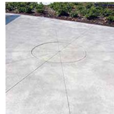
S4 - Saw Cut Concrete
