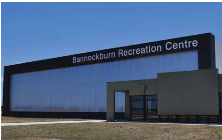
Bannockburn Recreation Centre
