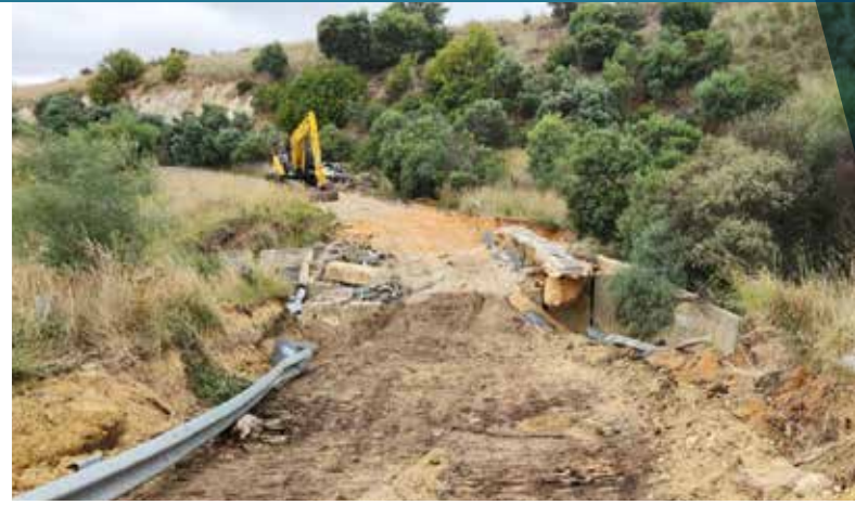
Linton-Piggoreet Road Bridge Reconstruction Preparation (shown above)
