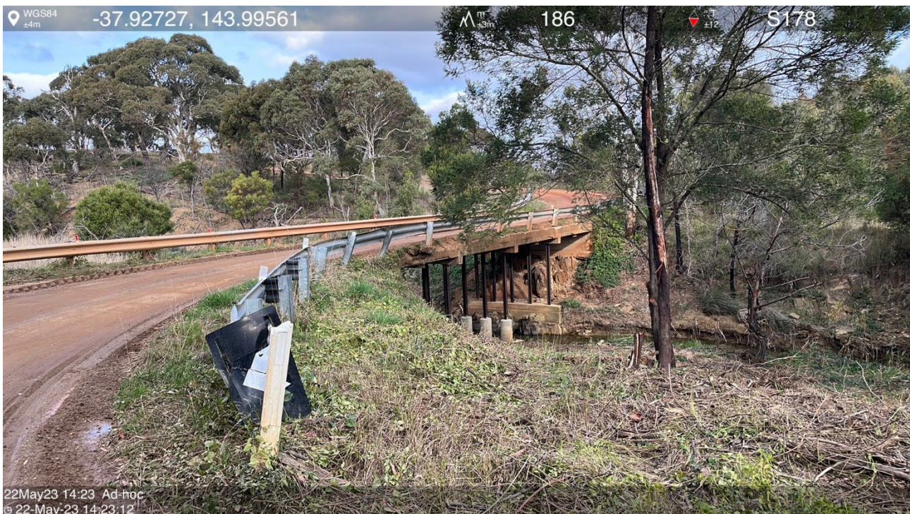
Photos of bridge showing damage to guardrail (vegetation recently cleared)
