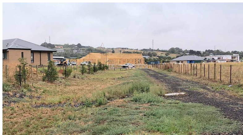
Figure 30: Southern access point from Vigneron Avenue.
