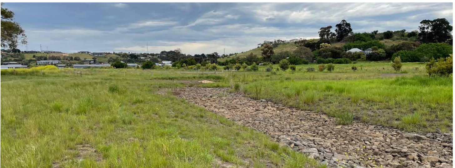
Figure 26: Clockwise from top left: mowed swale drain, stormwater retention wetland, and rocked swale drain.
