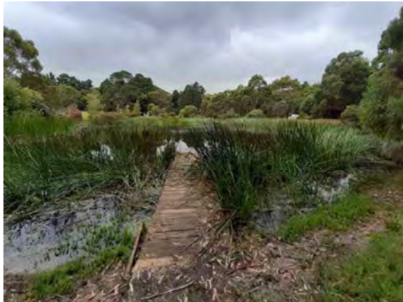
Jetty at Brewery Dam
