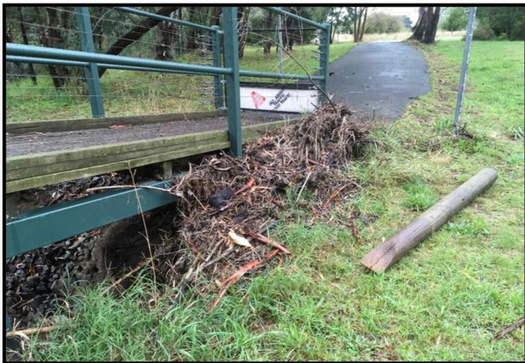
Flood debris build- up – refer above and below
