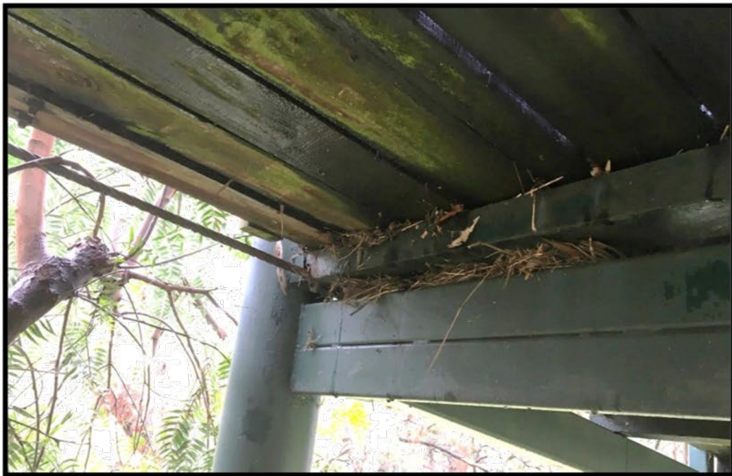
South abutment/ walkway: flood debris caught under deck indicating height of flood waters. Note deterioration and moss/ growth underneath planks.
