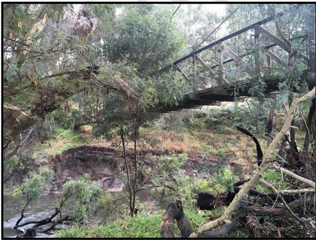
Profile views- note flood debris and vegetation growing next to and through structure- refer above and below
