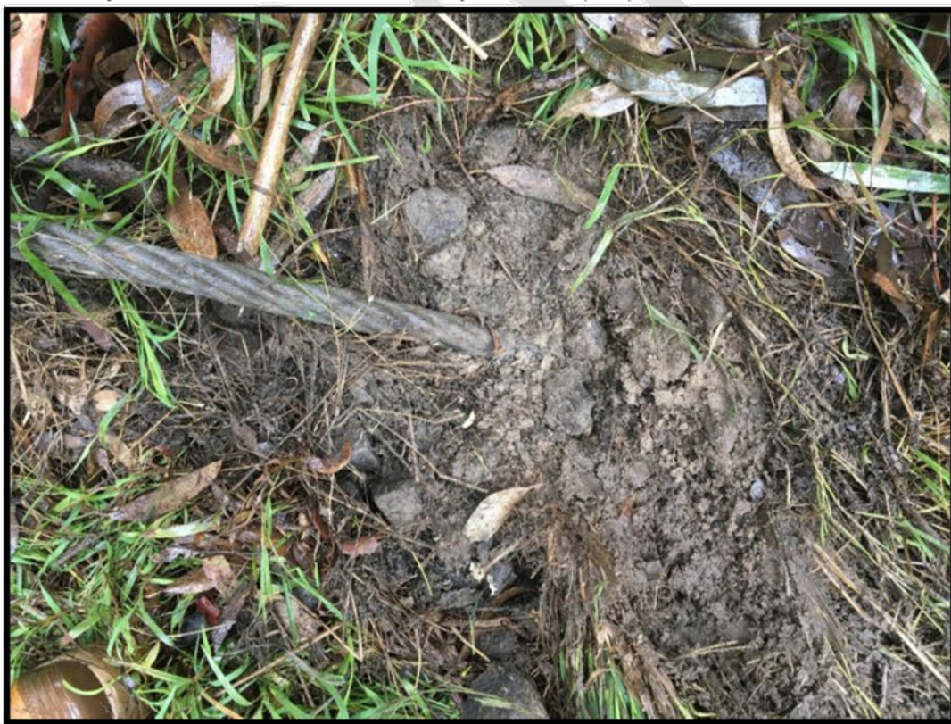
South- Catenary cables assumed to be directly embedded into concrete pad- note absence of adjustment mechanism and durability concerns (rust) - refer above and below
