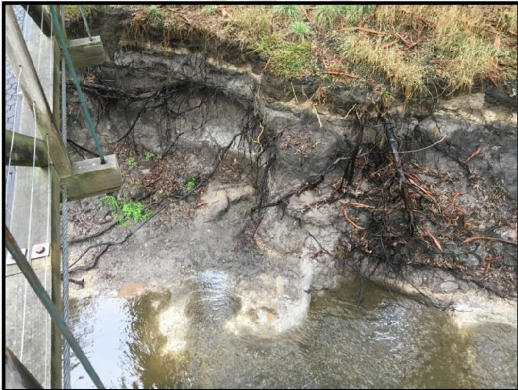
Significant scour to waterway does not affect bridge structure at this stage. To be referred to catchment authority for repairs
