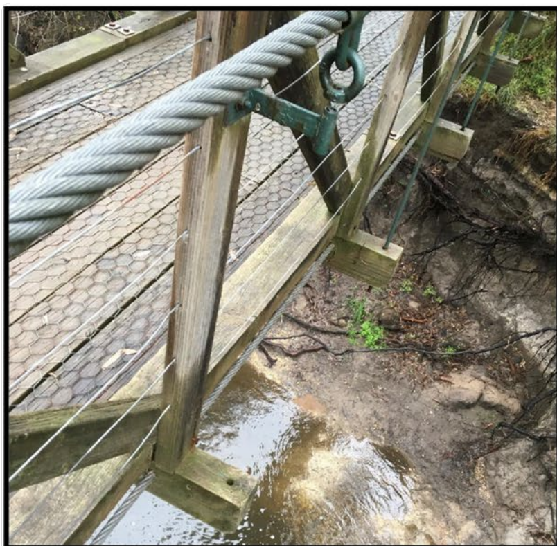
Missing suspender/ dropper
