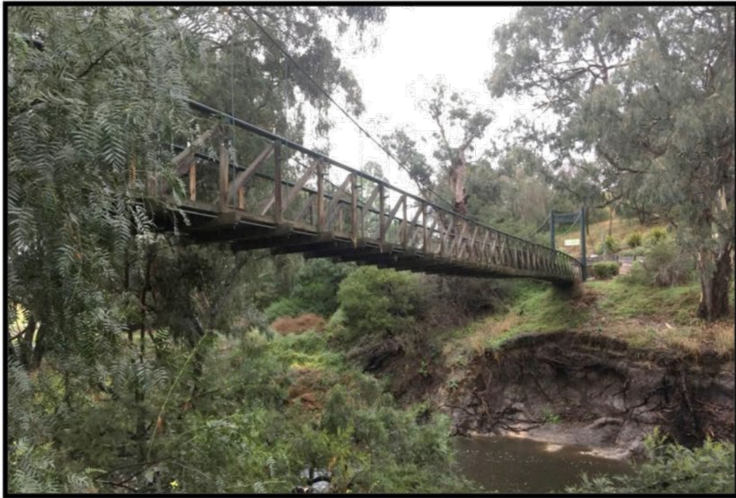
Profile views- note flood debris and vegetation growing next to and through structure- refer above and below
