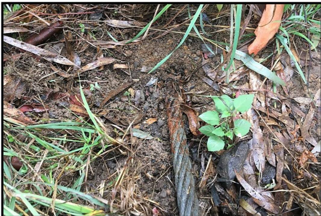
South- Catenary cables assumed to be directly embedded into concrete pad- note absence of adjustment mechanism and durability concerns (rust) - refer above and below
