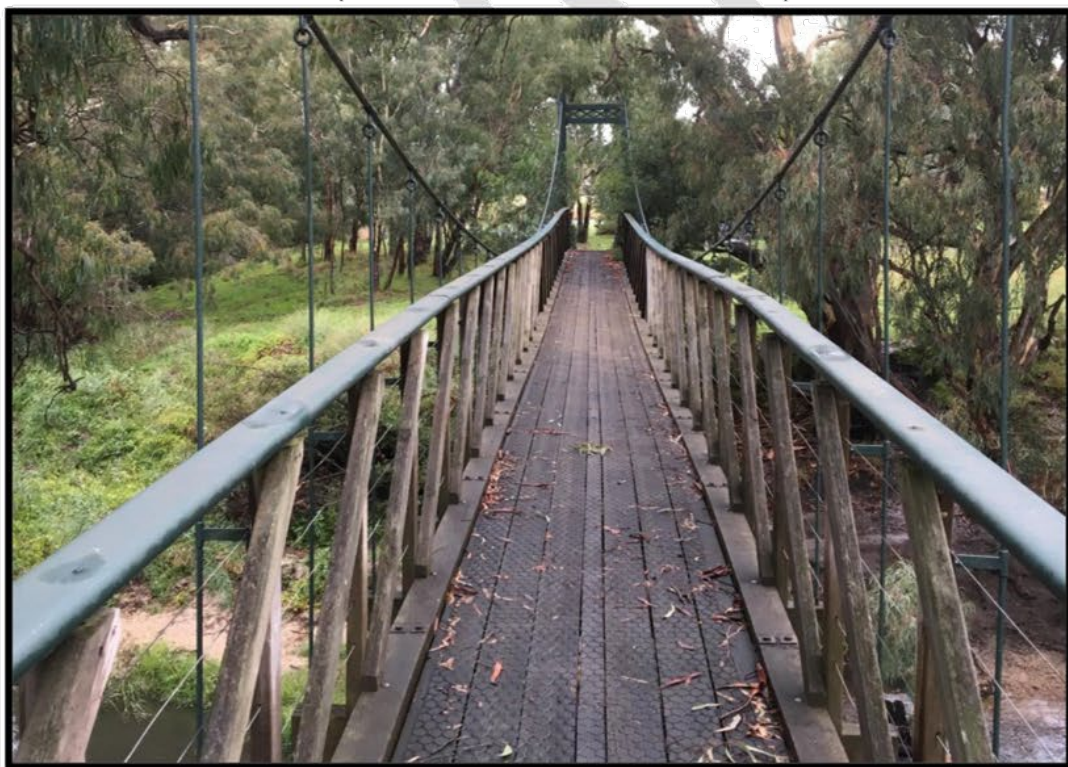
Deck is noticeably twisting towards upstream
