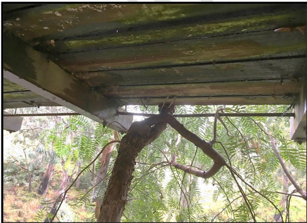
South abutment: tree growing under structure and through cable/ railing. Note deterioration, mould, lichen and moss underneath timber planks and beams
