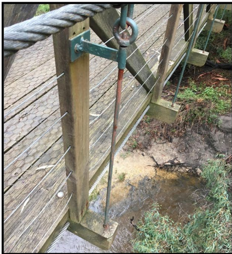
Example of corrosion to droppers
