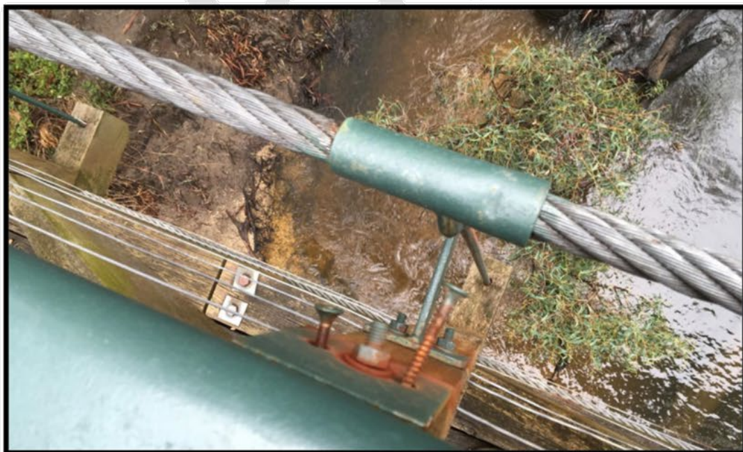
Example of corrosion and loosened fixings
