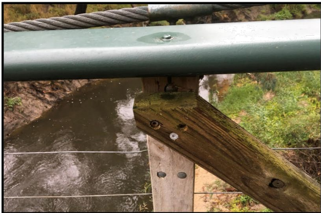
Guardrail deterioration and replaced fixings
