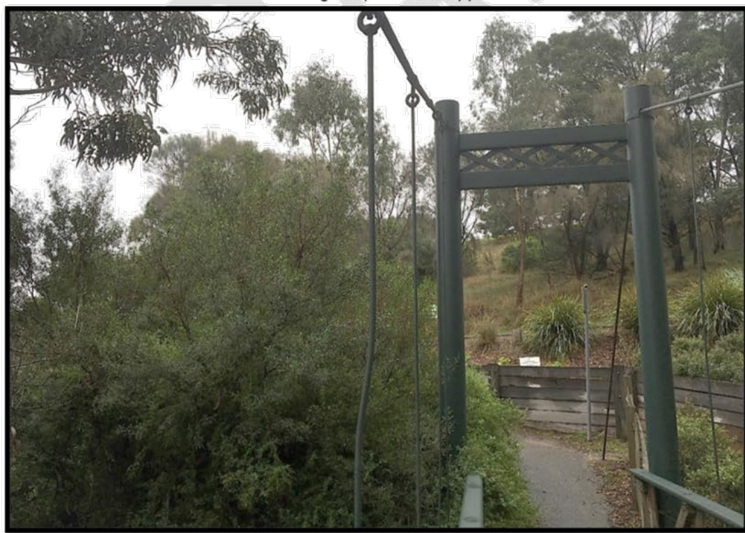
Example of bent droppers/ suspenders
