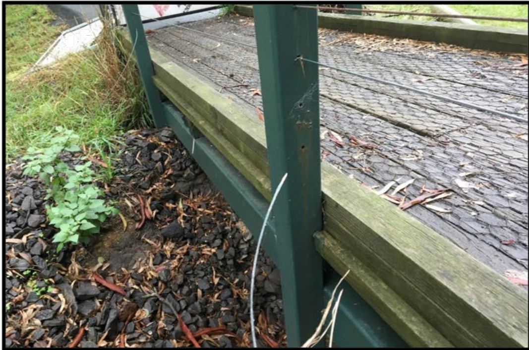
Broken strands of non-compliant horizontal wire fence
