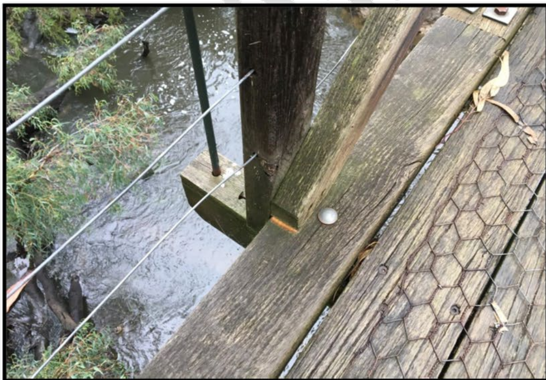
Signs of movement at deck/ railing joint
