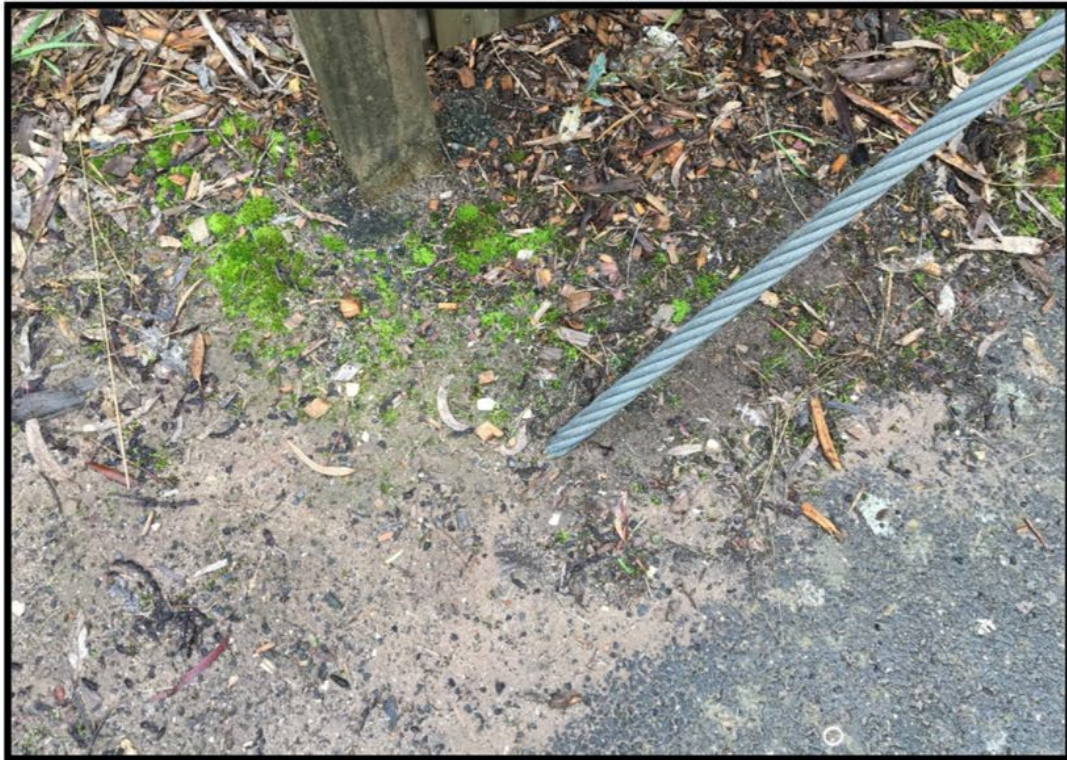
North- Catenary cables assumed to be directly embedded into concrete pad- note absence of adjustment mechanism and durability concerns - refer above and below
