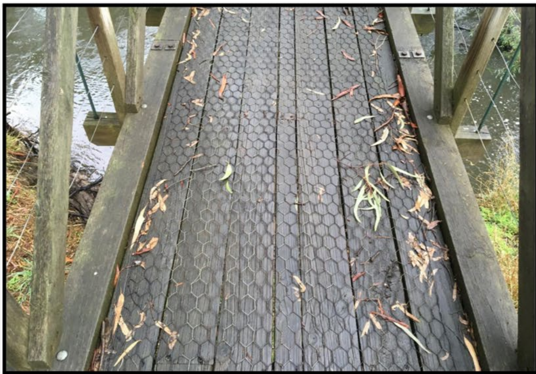
Non-compliant "chicken wire" installed on deck planks
