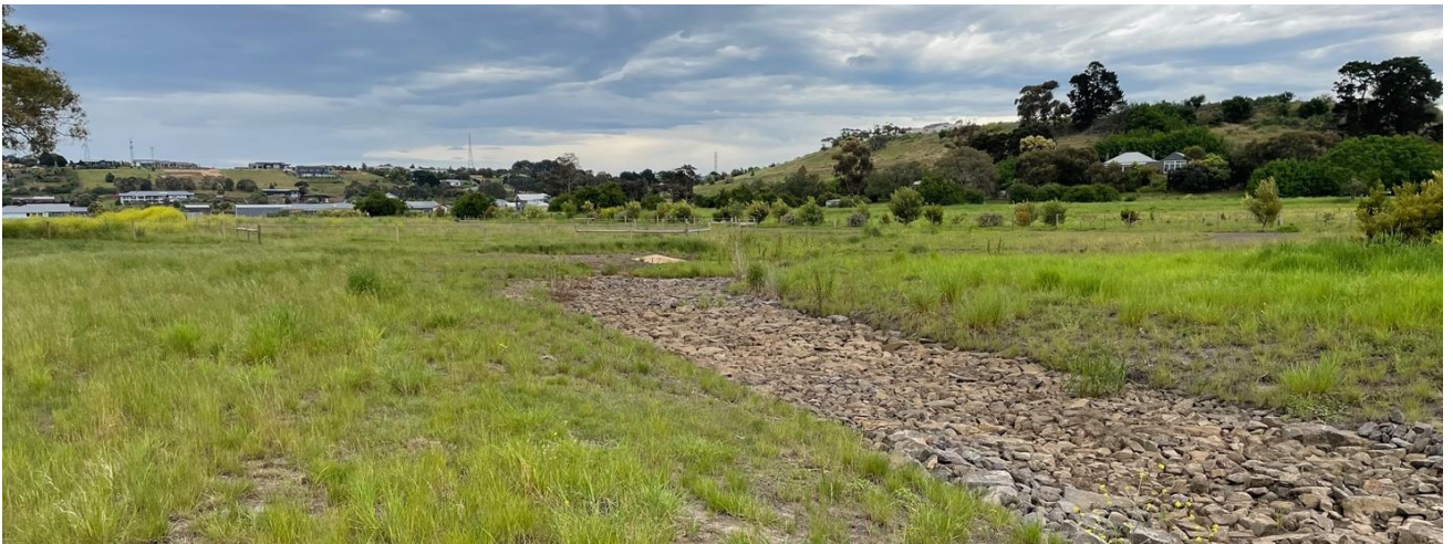
Figures 6-3, 6-4, 6-5: Clockwise from top left: mowed swale drain at the southern access point, stormwater retention wetland, and rocky swale drain installed to capture stormwater run-off from the adjoining Riverstone development 383940
