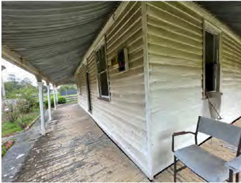
Figure D4. Pre 1884 house showing the timber weatherboard clad walls, the window and door openings with broken window panes, and the self supporting convex corrugated iron verandah roof cladding, which is supported on classical timber posts at the outside edge of the verandah.
