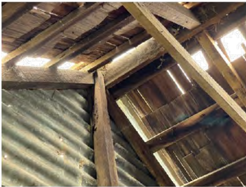
Figure D10. Interior view of the roof structure and the underside of the timber paling roof shingles.
