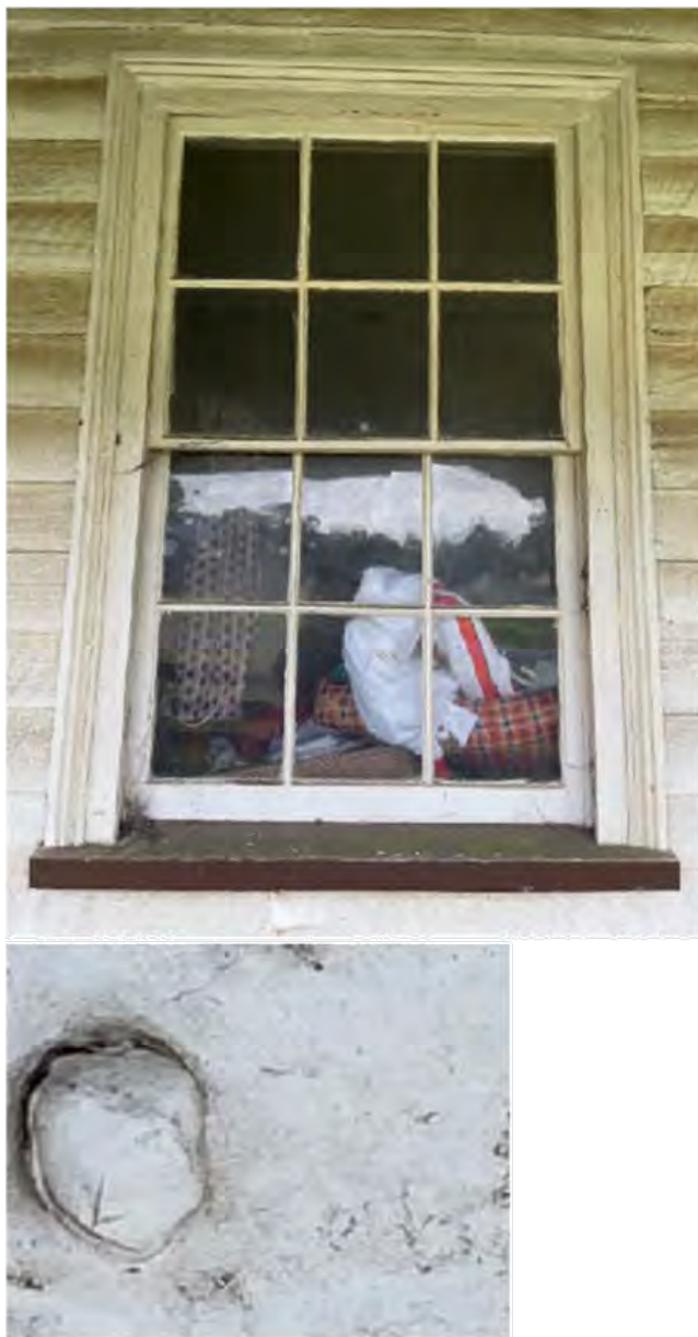
Figure D3. Window details on the pre-1884 house showing the 12 pane double-hung timber sash, moulded timber window frames, and 'chew' marks on the upper weatherboards and an example of the early nails used to fix the early weatherboards.
