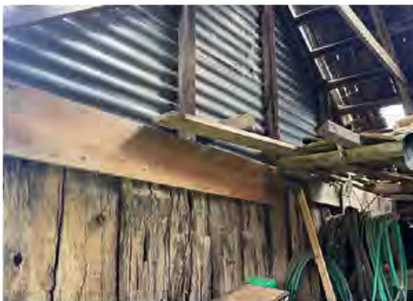
Figure D11. Interior view of the south elevation of the former stables and buggy shed, showing the timber structure with very large timber adzed slabs forming the wall. This building is likely to be contemporary with the pre 1884 house.
