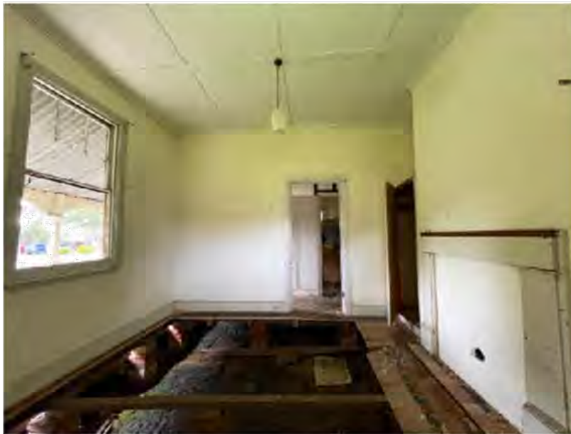
Figure D5. Interior view of a front room in the pre 1884 house showing the 'Regency' styled timber fireplace surround on the right, 'missing floor boards' in the centre, cement sheet/masonite ceiling and wall cladding and damaged window glazing on the left. Note. If the existing cement/masonite internal wall and ceiling linings are removed care must be taken to record in photographs and measurements of the linings behind them. The original linings are likely to be timber boards with wall paper over them as noted in the 1905 valuation as 'wooden partitions, papered'.
