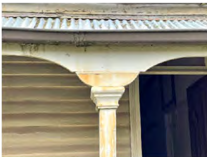
Figure D7. Detail view of the timber valance, capital and chamfered post. The quad gutter is a later addition as it would have been galvanised iron ogee profile.
