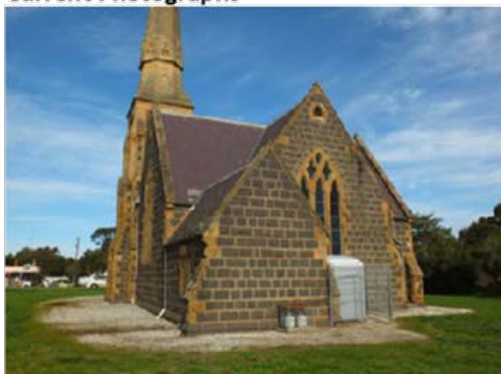
Rokewood Presbyterian Church, rear (north) elevation showing projecting vestry.
