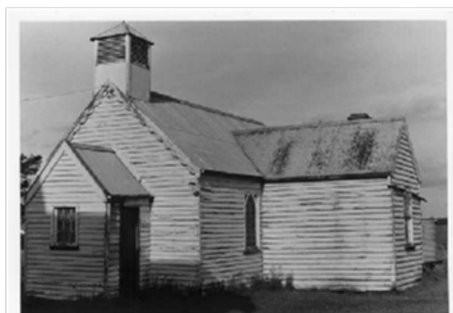
Christ Church (original church building), 30 November 1968. Source: J.T. Collins, La Trobe picture collection, State Library of Victoria, image jc011977.
