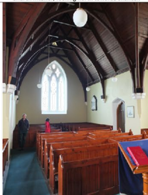
Church interior, looking south.
