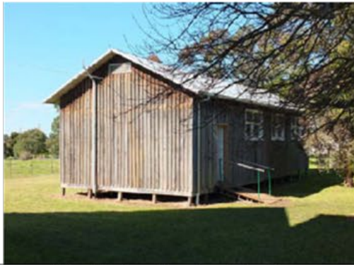
Church Hall, north and west elevations.
