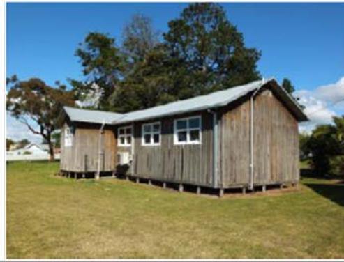
Church Hall, north and east elevations.
