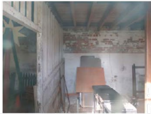
Interior, police stables.
