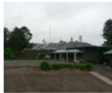
Woolbrook homestead from the north west
