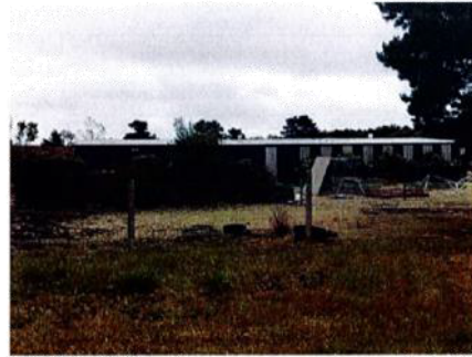
View of subject site's attached shed from Steddy Road
