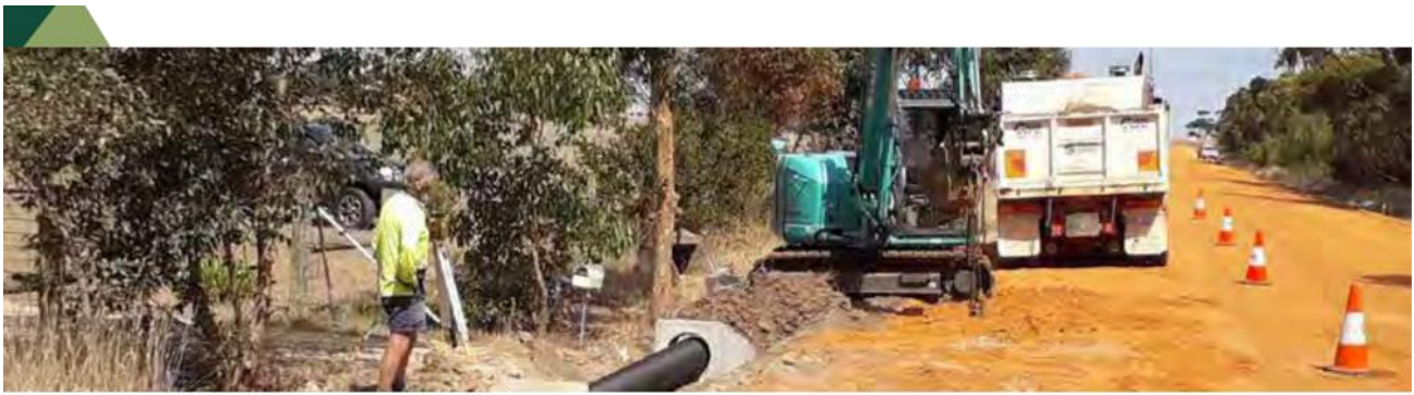
Tall-Tree Road construction works.
