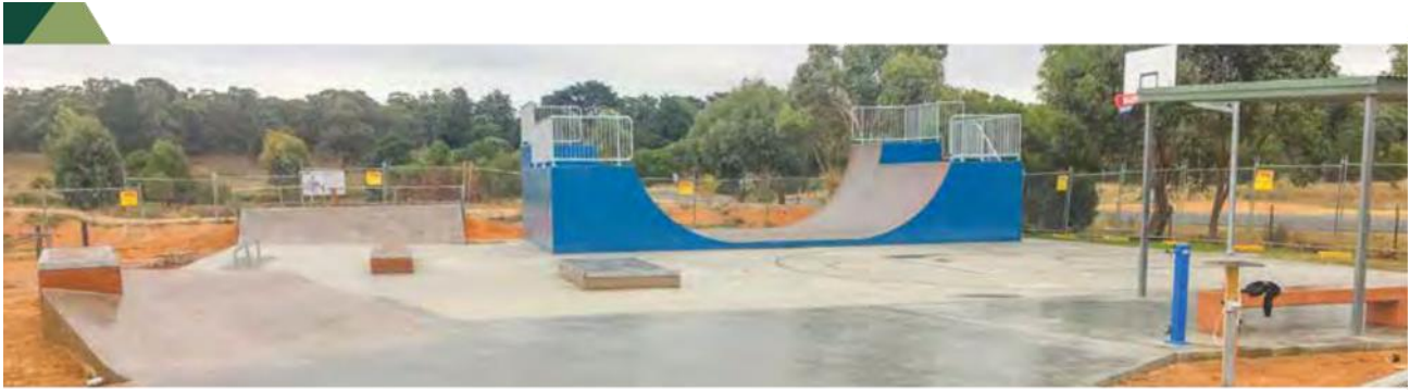
Smythesdale Skate Park during construction.
