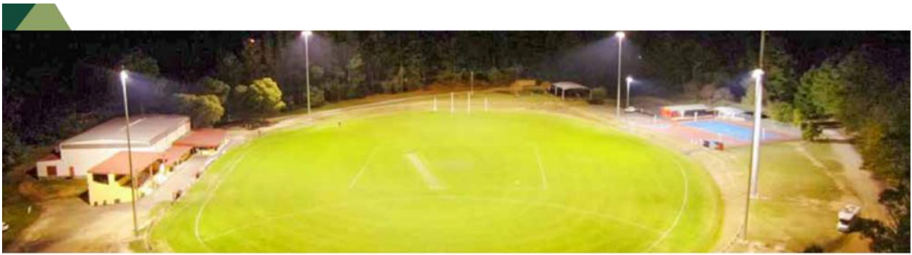
Linton Oval Lighting.
